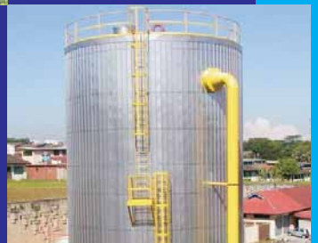
Hospital UKM, Cheras Capacity: 12,950RTh, Size: 27' Dia x 56' H
