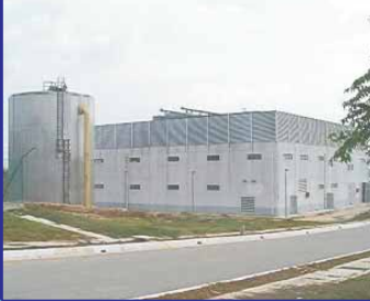
Multimedia University, Cyberjaya Phase 1 Capacity: 11,000RTh, Size: 29' Dia x 41' H
