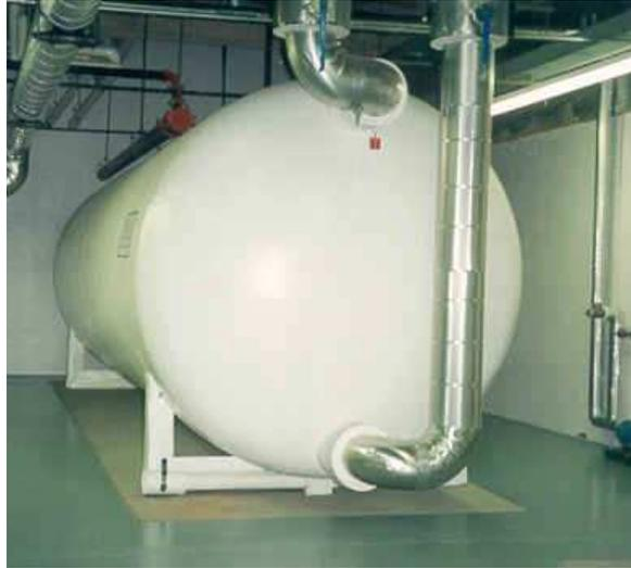
*Cryogel Ice Ball Thermal Storage Tank*
