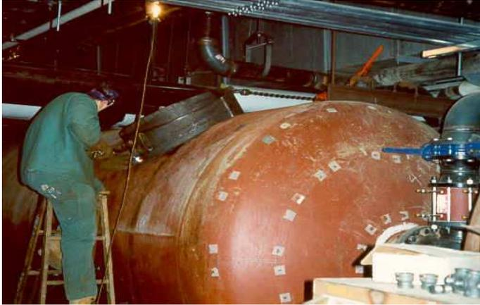
Ice is produced over a period of 8 hours during off-peak night hours. Chillers operating at a capacity of 250 tons, cool Wintrex heat transfer fluid supplied by Houghton Chemical of Boston to an average temperature of 22.2°F. That cold fluid is then circulated through the storage tanks and Ice Balls to make ice and store energy until it is needed during the afternoon when air conditioning loads peak.
