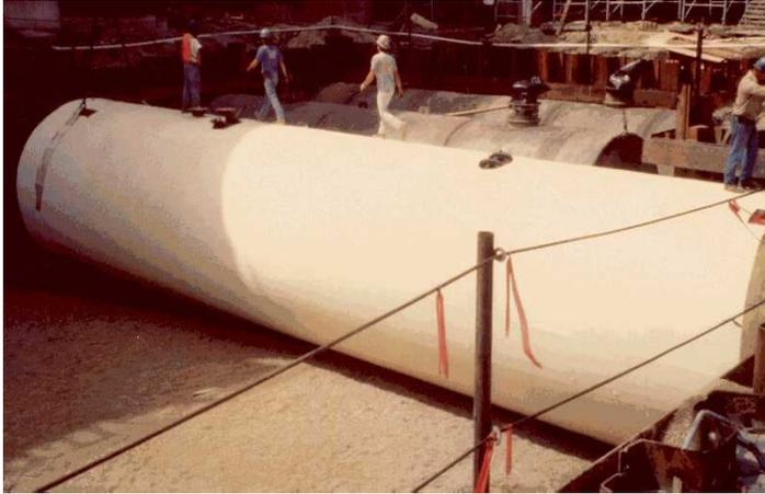
First of four tanks set on sand base.
