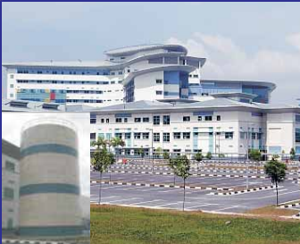
Hospital and College, Sungai Buloh Capacity : 9,400RTh, Size: 26' Dia x 43' H
